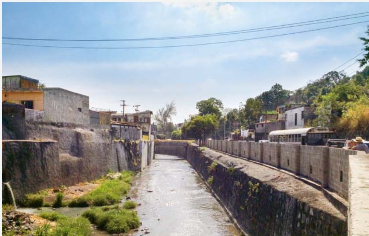
Our ECA study for San Salvador found that further improving river bank reinforcements such as these can significantly reduce damage from flooding and protect vulnerable houses.
