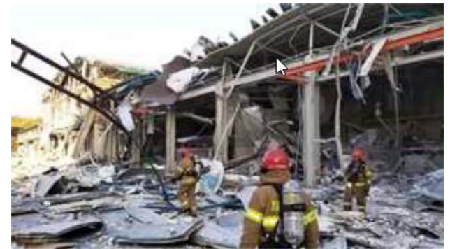
Explosion of an outdoor hydrogen tank at a water electrolyzer plant coupled with a solar photovoltaic power system (May 23th, 2019) → 2 fatalities and 6 injuries (USD 30-40 million damage)
