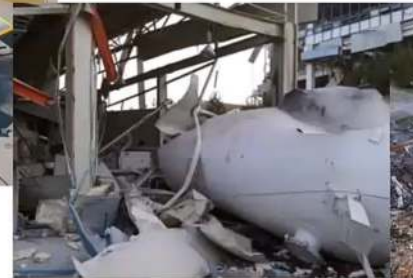
South Korea, 2019 Hydrogen tank explosion
