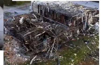
Illinois, USA, 2019 Hydrogen blast at AB Speciality Silicones factory
