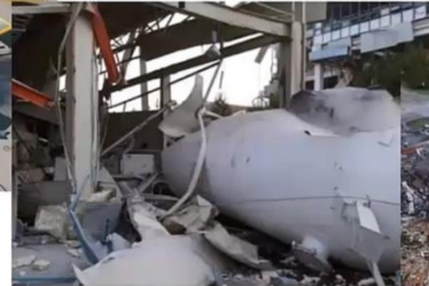
South Korea, 2019 Hydrogen tank explosion
