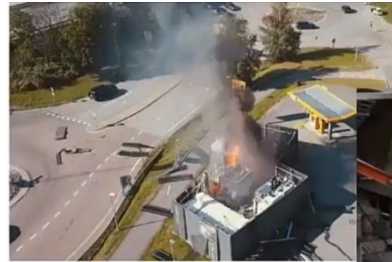
Norway, 2019 Hydrogen fuelling station explosion
