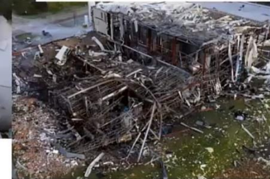
Illinois, USA, 2019 Hydrogen blast at AB Specialty Silicones factory
